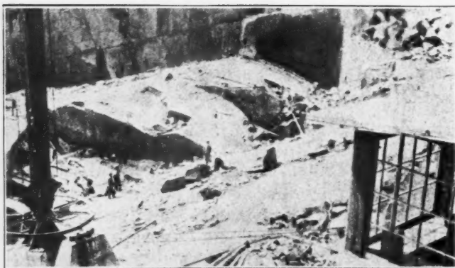
Quarry Floor Showing Present Working Ledge
